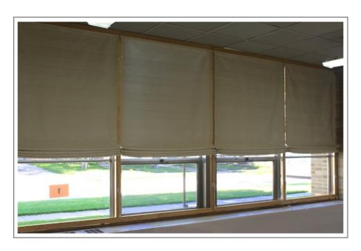
The shades will provide an **R-Value of 6.39**, stop the chill of cold air from coming off the windows, and keep the warm air going into the classroom where it will have the greatest benefit. *This one wall section now has the highest insulation value of the entire building's exterior.*
